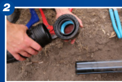
2 Remove the O-ring, then the split ring, collet and nut, then re-assemble the fitting and it is now ready to use.
